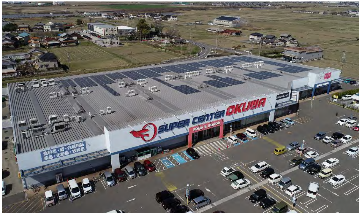
Solar power plant in operation at Super Center Yoro Store since Mar. 1, 2023
